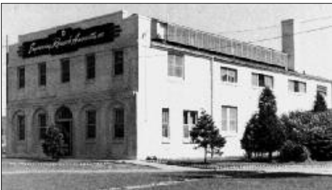
Engineering Research Associates building, located at 1902 W. Minnehaha Ave. From the collections of the Dakota County Historical Society.
