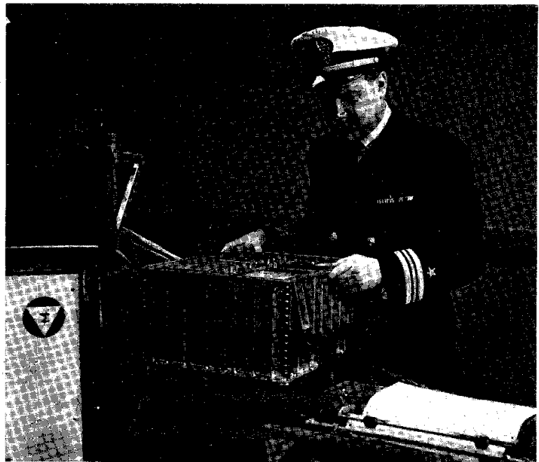
UNIVAC DIGITAL COMPUTER will play key role in Project A-New integrated ASW avionics system which Naval Air Development Center is assembling for installation on YP-3A. Flight evaluation of the experimental system is scheduled to begin early next year.
