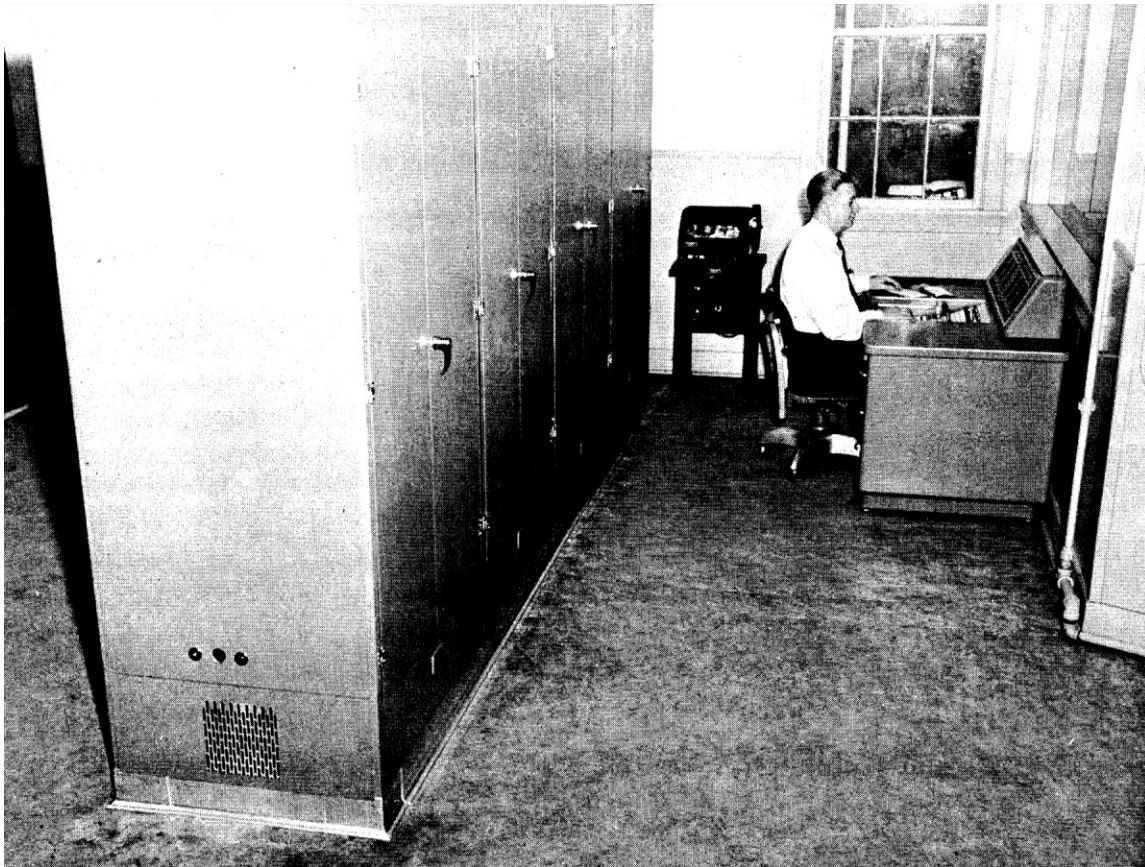
Railroad Car Weighing System
