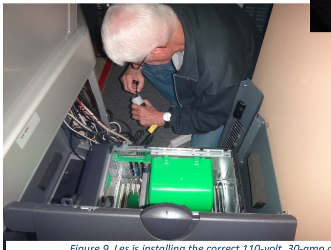
Figure 9. Les is installing the correct 110-volt, 30-amp connector.
