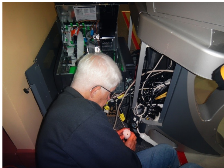
Figure 7. Les Nelson examining the power connections.
